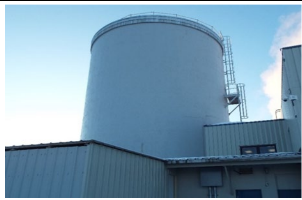
Photo 4: Exterior view of structure containing the SM-1A VC
