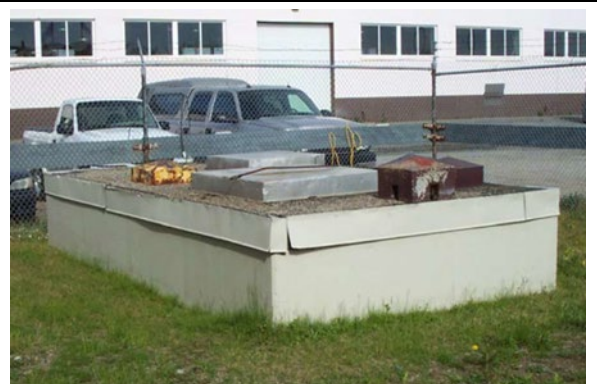
Photo 6: Well No. 11 Pump House
