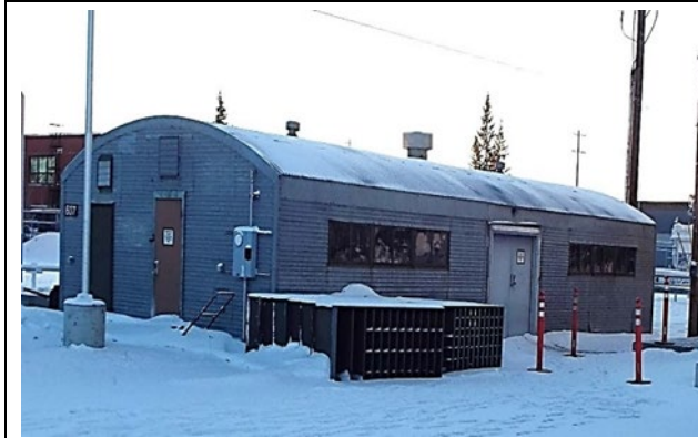
Photo 3: Building J-5 (also known as Building 607)
